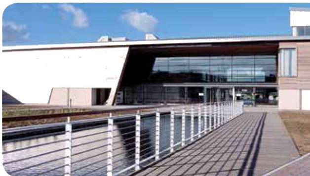
National Maritime College of Ireland (NMCI)
